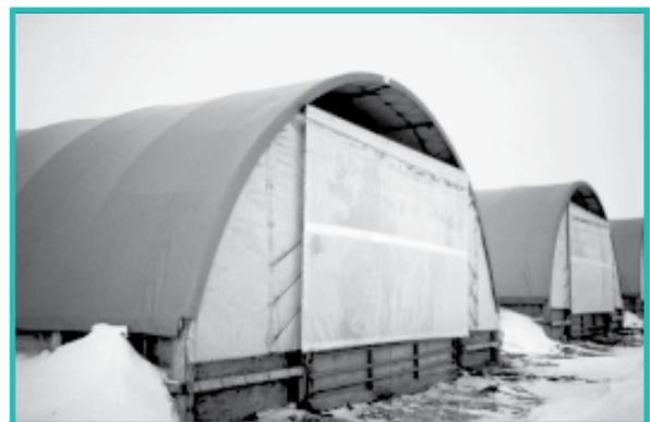
Figure 5. Cloed end of hoop during cold weather. Source: Based on Figure 13, Hoop Structures for Gestating Sows, AED44.
