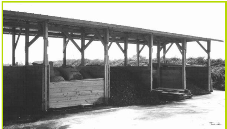
Bin composter showing typical features such as concrete pad, wooden bins with drop boards, and a roof. Adapted with permission from Stettler D. Livestock and poultry environmental stewardship curriculum: mortality management. Lesson 51. Ames, IA: Midwest Plan Service. 2001.
